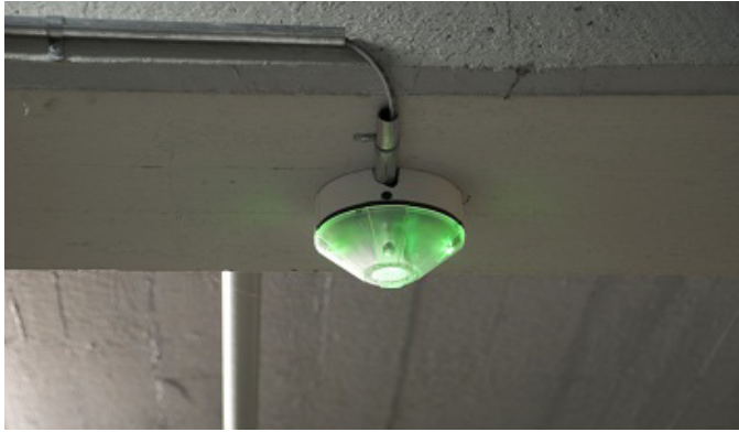
Fig. 37: Lowered sensor installation
