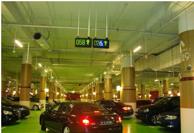
Fig. 37: Lowered sensor installation
