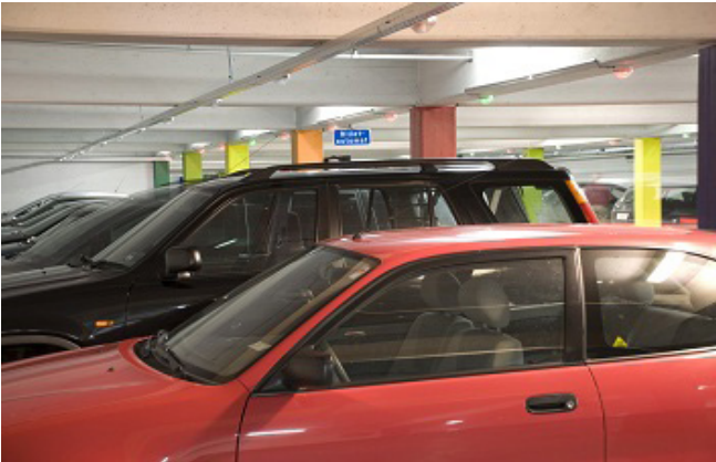
Fig. 35: Sensors mounted on cable tray
