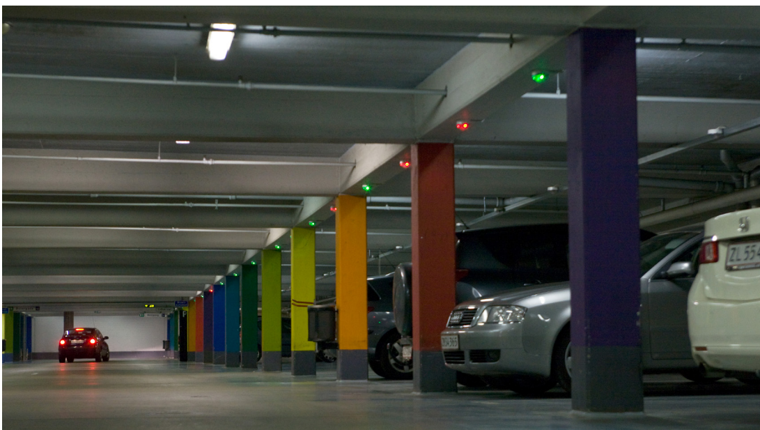
Fig. 19: Driveway with external indicator lights providing a clear view
