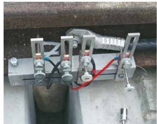
On site testing
