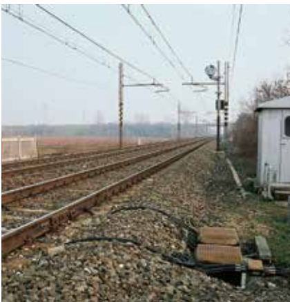
Signalling and traction current connection to manganese steel cast exchange units
