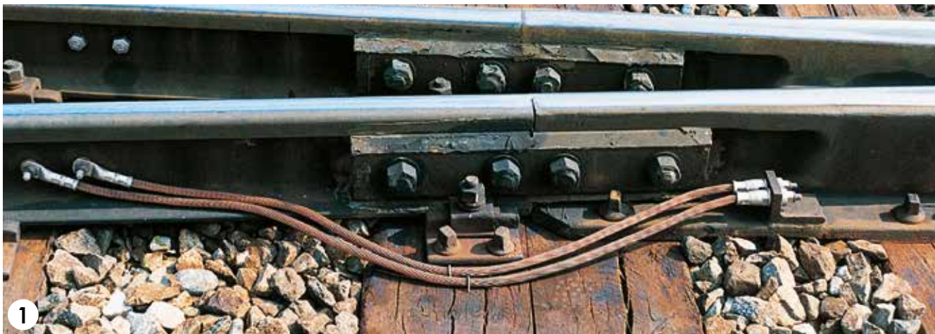
1) Example of electrical connections using a low stranded conductor to provide electrical continuity on cast manganese steel crossovers.
