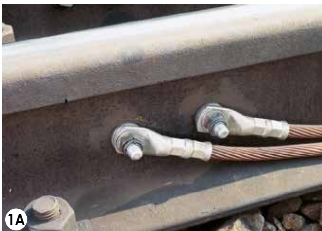
1) Example of electrical connections using a low stranded conductor to provide electrical continuity on cast manganese steel crossovers.
